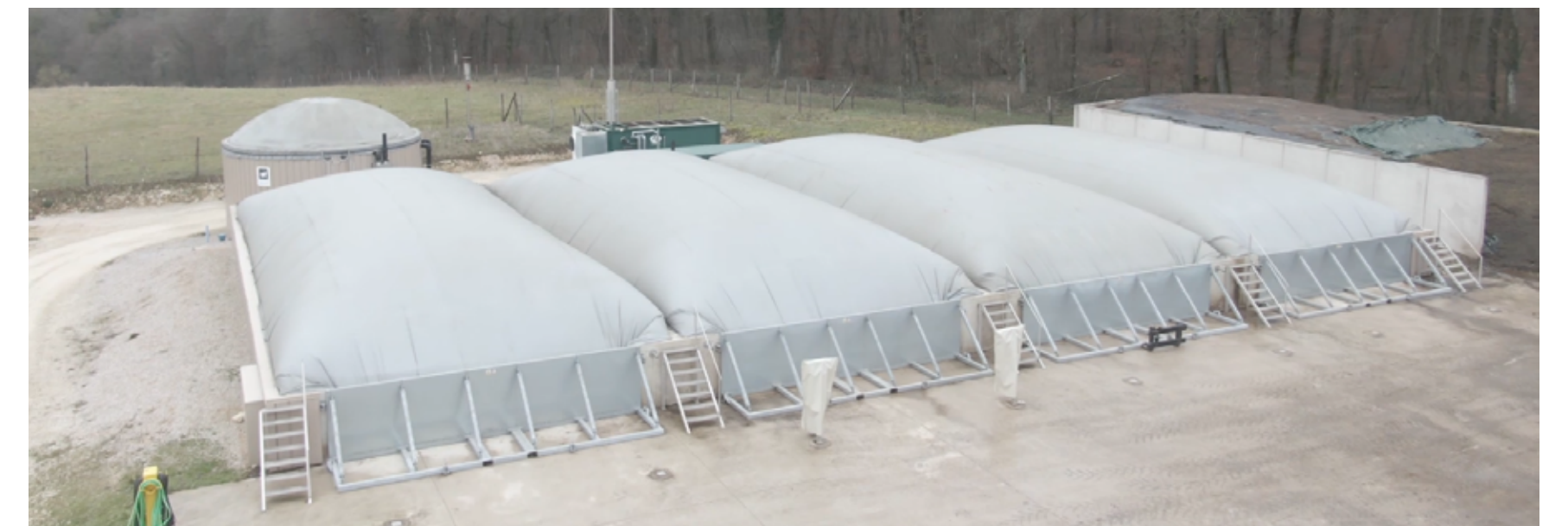
Figure 4: An example of a dry anaerobic digestion system for the production of biogas (Joly biogas plant in France)
